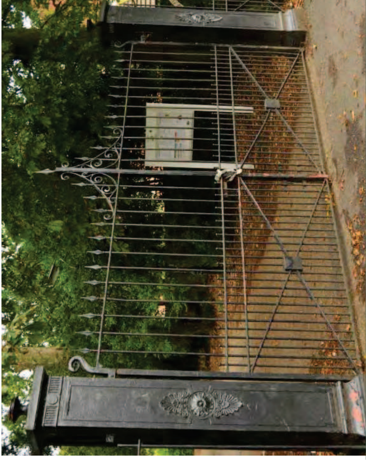
Iron boundary railings and gates to Barra Hall Park
